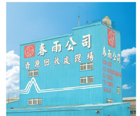
廢酸回收工場 Acid Treatment System
